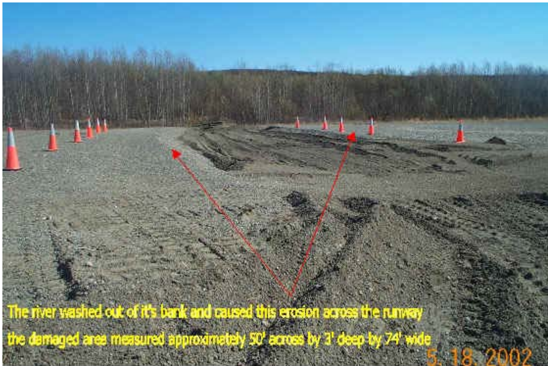
Photo 1: Red Devil airport erosion caused by 2002 ice jam flood. Area measures 50 feet across by 3 feet deep by 74 feet wide. Photo courtesy of DHSEM, 2002.
